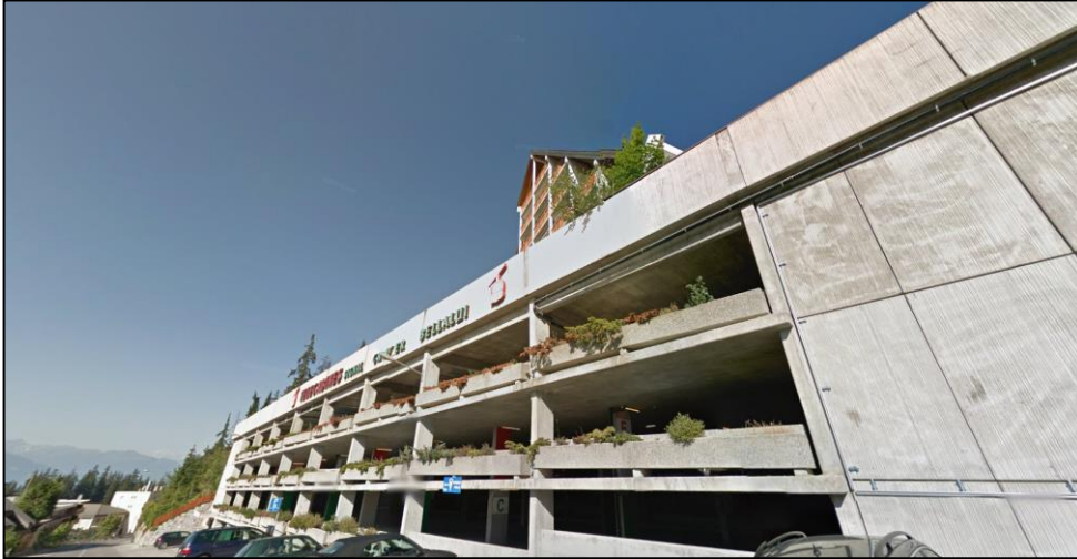
Parking Signal – Rénovation total – Crans-Montana (Façade Sud)
